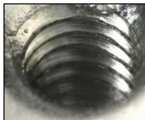
Condition of good internal threads
